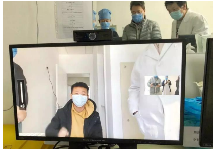
Avaya engineers installing remote consultation video systems for isolation wards.
